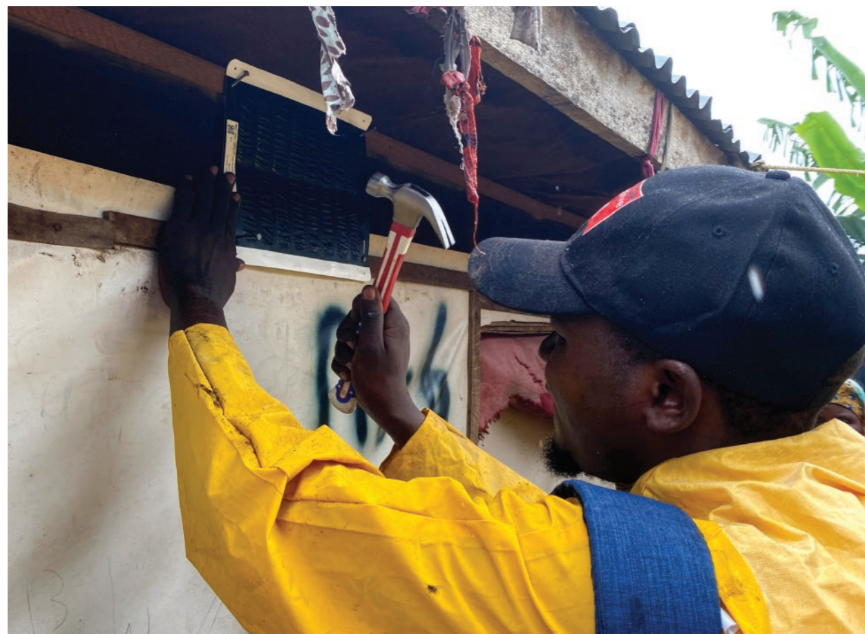
Installing the attractive targeted sugar bait during the trial in Nigeria.
